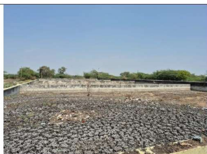
Sludge drying bed with negligible amount of sludge
