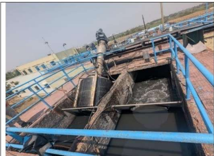
One of the screen chambers without rotating screen
