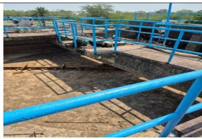
Grit chambers with defunct scraper mechanisms
