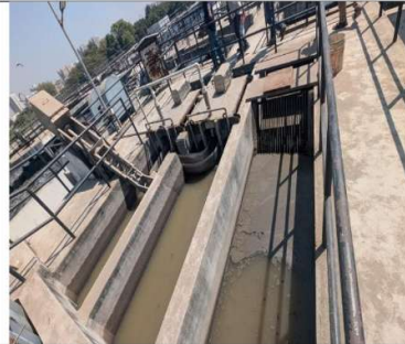
One of the grit chambers not in operation
