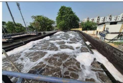
White foam in aeration tank indicating inadequate MLSS in aeration tank
