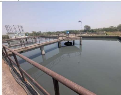
two out of four aerators in aeration tank was defunct
