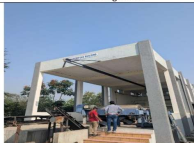
Centrifuge seems not operated regularly and sludge drained on open land
