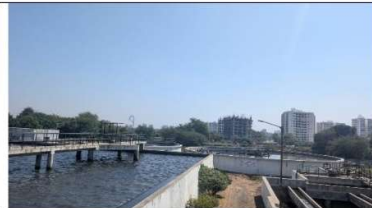
Black colored Aeration tank
