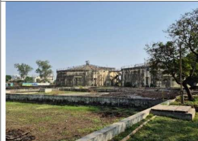
Empty sludge drying bed with vegetation.
