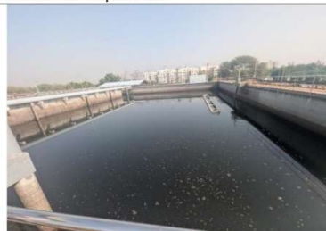
SBR in settling mode
