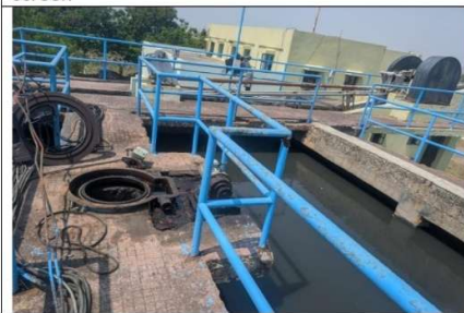
Grit chambers with defunct scraper mechanisms
