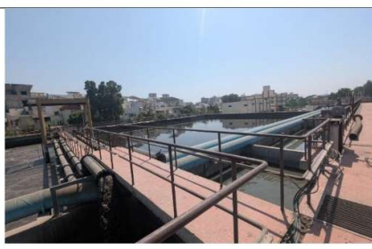
SBR under settling mode
