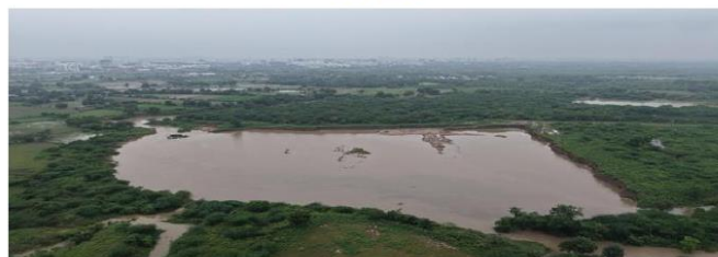
After work Lake Formation (Picture dated 05/09/2025)
