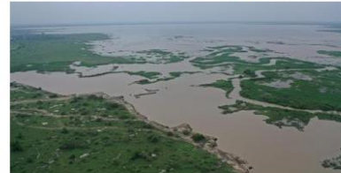
After work Lake Formation (Picture dated 05/09/2025) 26 | 49
