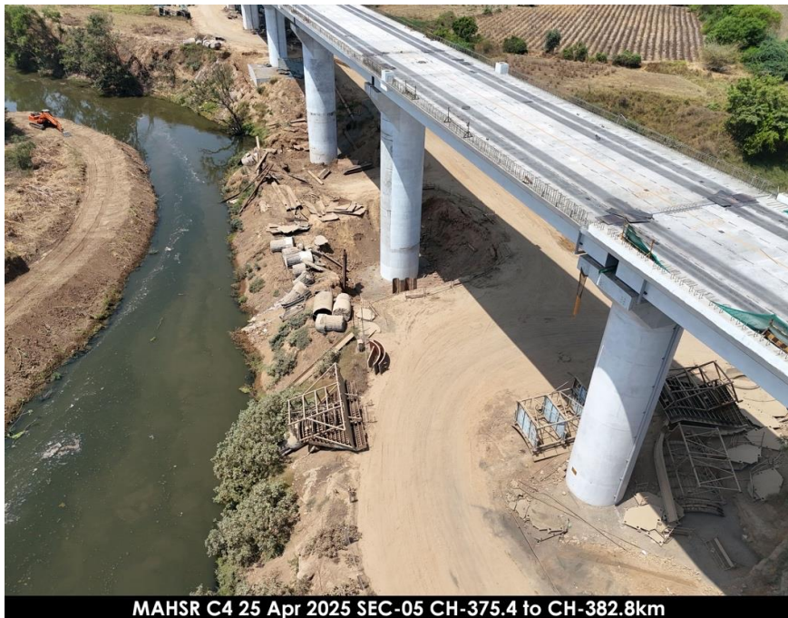
MAHSR C4 25 Apr 2025 SEC-05 CH-375.4 to CH-382.8km
